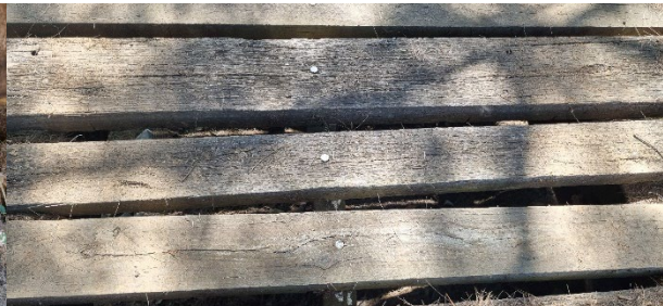
Plate 5.4 Photo of decking gaps on Durbin Street Bridge
